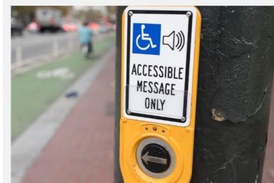
Accessible Pedestrian Signals
